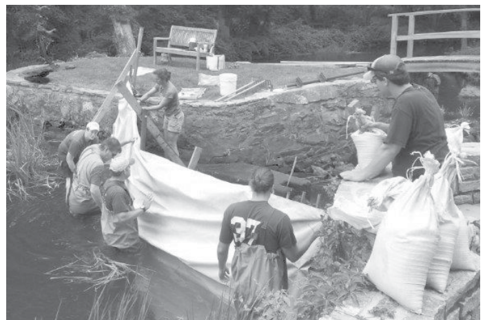
Workers from the Nature Conservancy and state DEEP spanned the spillway with an impervious tarpaulin anchored with sand bags. The pond drained through a second spillway, at far left.
